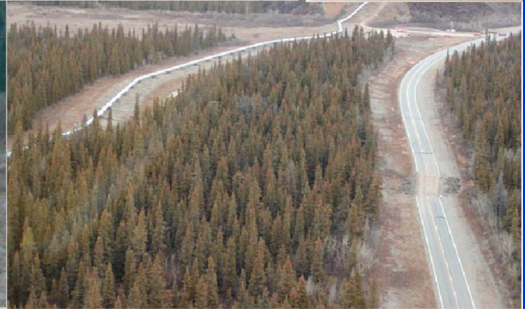
Locality 3 on Map. Aerial view of the Trans-Alaska Pipeline and Richardson Highway, looking north. Rupture along the fault resulted in approximately 2.5 meters (8 feet) displacement of the highway, with the north side moving east relative to the south side. Photo by Patty Crow, DGGS.
