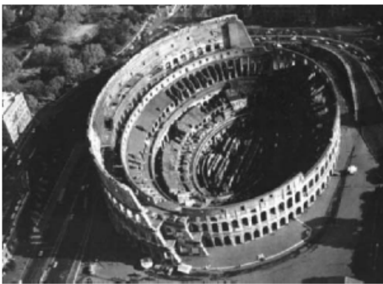
FIGURE 5 The Roman Colosseum: the missing half of the outside wall collapsed in an earthquake in 1349 (Guidoboni, 1994).
